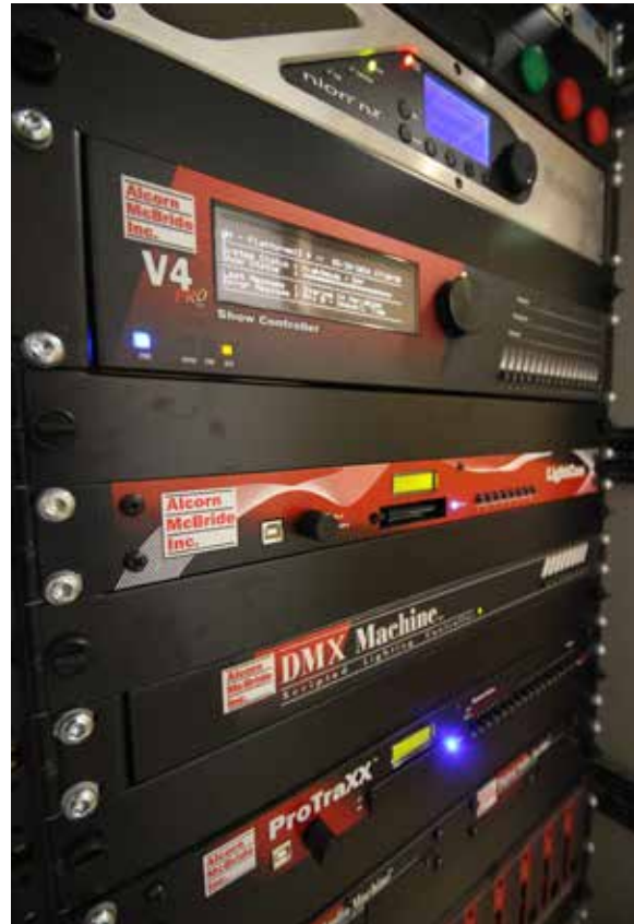
A rack of AV equipment controls is the heart and brains of an attraction. All photos courtesy of Alcorn McBride.
